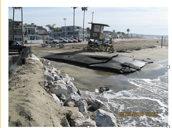
Figure 3. 20 th Street (Newport Beach Public Works)
